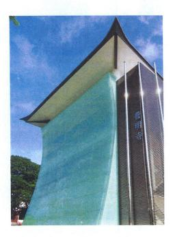
Digital glass printing is no longer traditional printing technique — texts and graphics are firstly transformed into computer processed data, then printed on glass by special inkjet printers or electronic printing machines without contact. Not only does it overcome the quantitative constraints of traditional printing methods, but it also leads to simpler and more stable printing process than screen printing or pad printing.
